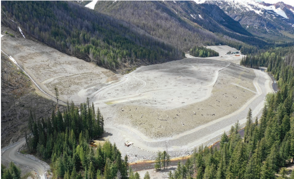
The reclaimed Holden Mine closure project in Washington state (photographed in 2019) is a great example of a sustainable mine closure. CREDIT: STANTEC
