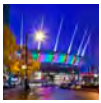
BC Place Vancouver, British Columbia Services: Architecture and Interior Design Prime Consultant: Stantec in association with Cannon Design (Turf & Seating)
